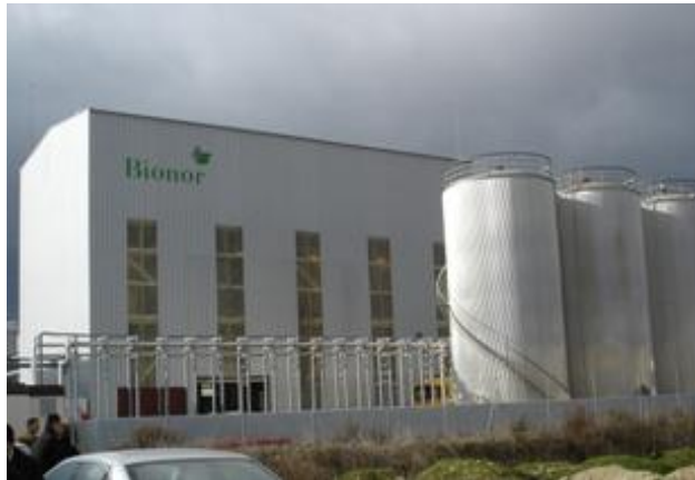
Biodiesel production plant of Bionor in Berantevilla
